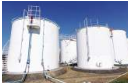
According to ExxonMobil, the dual imager IntelliRed remote gas detection system is a step forward in mitigating operational risks while improving reliability and ease of use. (Photo: Akiyoko/Fotolia)
