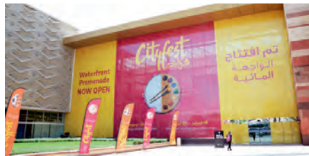
Coopers fire and smoke curtains are used to protect Dubai Festival City Mall
